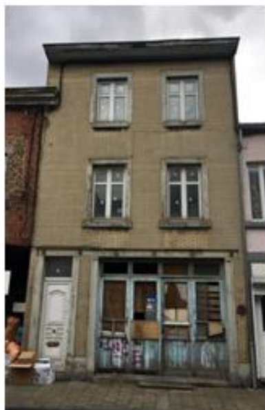
B: Heavy renovation needed
